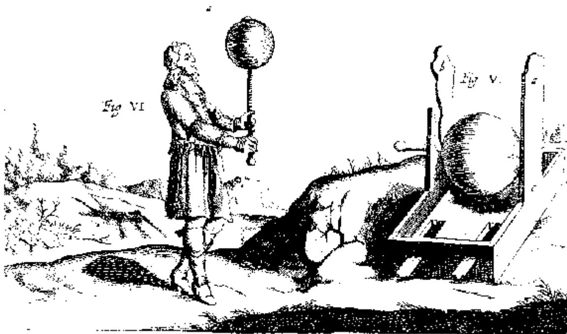
**Fig. 1.6.** Otto von Guericke constructed the first electric machine which included a sphere of sulphur with an iron axle. When rotating and rubbing the sphere it generated static electricity. (Guericke, 1672).
